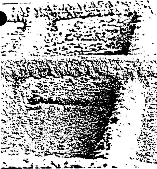
Fig. 8.11—Overspray on reinforcing bars at the top of a band of shotcrete. If the overspray is permitted to harden, and remain on the bars during the next application of shotcrete, it will be impossible to fill behind the bars with good shotcrete. Large hollows will remain in the wall, promoting cracking and moisture penetration.
