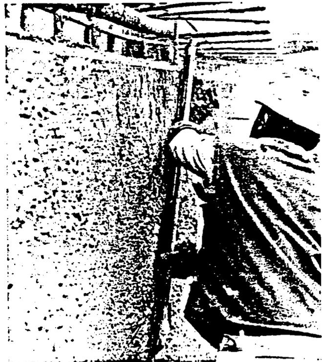
Fig. 8.12—Screeding excess or overgunned shotcrete leaving rough textured finish
